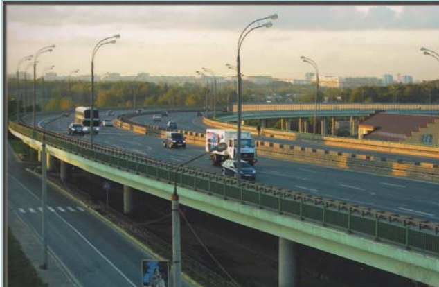
• RUSSIA, MOSCOW -- Vidnoe Viaduct expansion joints
