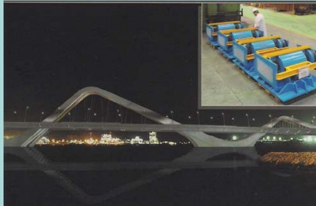
• UNITED ARAB EMIRATES, ABU DHABI -- Sheikh Zayed Bridge seismic isolators, viscous dampers, fuse restraints
