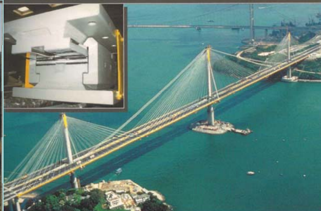
• HONG KONG -- Ting Kau and Tsing Ma Bridges pot, spherical and cylindrical bearings with uplift capacity, lateral restrainers
