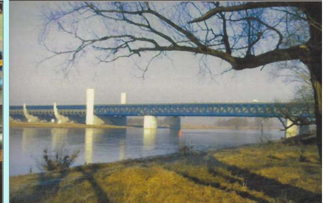
• GERMANY, MAGDEBURG -- Water Bridge shock transmission units
