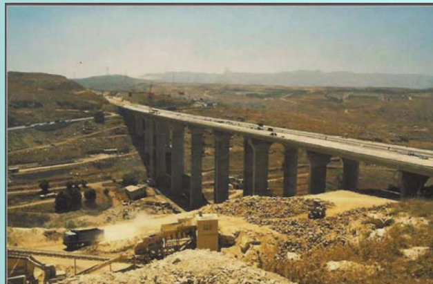
• LEBANON -- Beirut - Sirian Border Highway expansion joints
