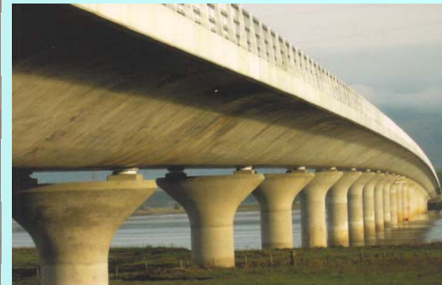
• U. K., KINCARDINE -- New Bridge pot bearings, expansion joints
