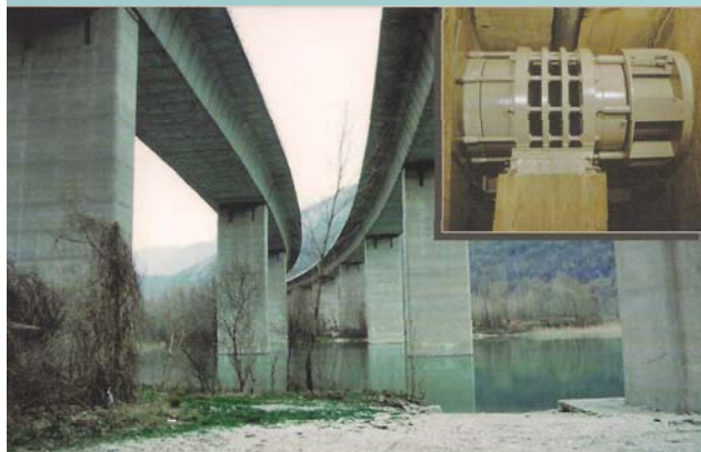
• ITALY -- Somplago Viaduct buffers, Europe's first seismically isolated bridge, 1974
