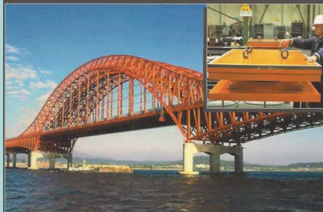
• SOUTH KOREA -- Bang Hwa Bridge spherical bearings
