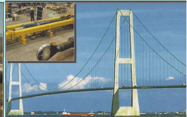
• DENMARK -- Storebælt Bridge shock transmitters 5000 kN, ± 1100 mm, spherical bearings
