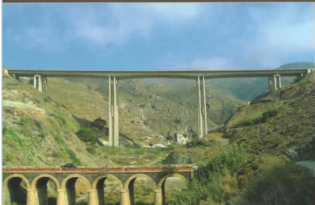
• SPAIN -- Alcazaba Viaduct, Autovia del Mediterraneo Albulon - Adra viscous dampers
