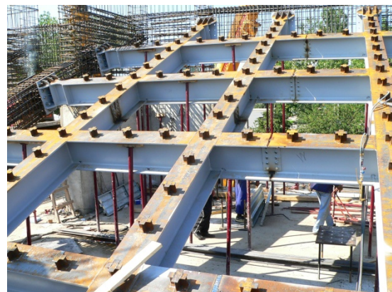
Figure 5. Steel Grid of the Sloped Floor
