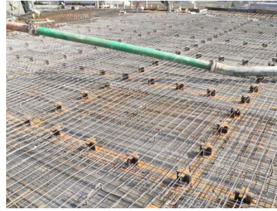
Figure 7. Rigid Connectors and Slab Reinforcement
