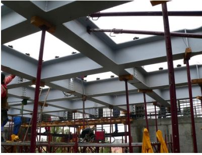
Figure 6. Steel Grid of the Horizontal Floor
